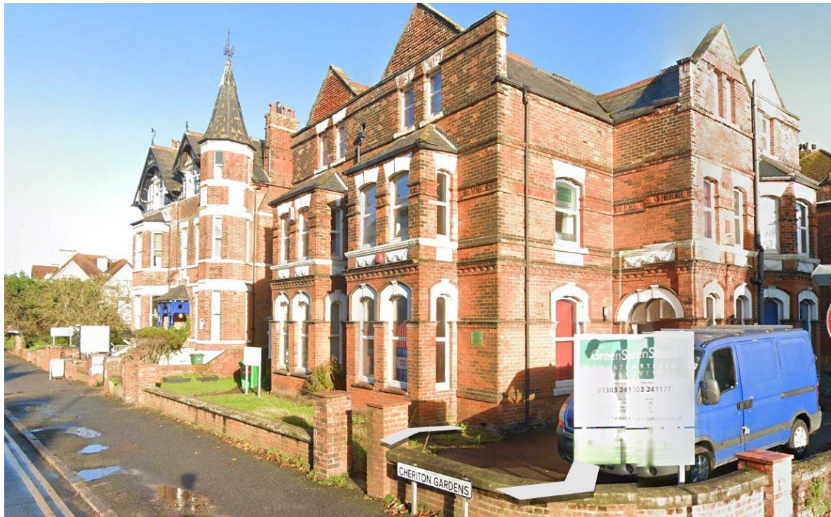
Plate 1. The site (looking north- Google Earth/Street View)
