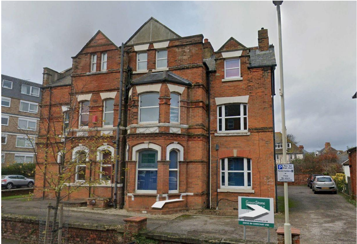
Plate 3. The site (looking NE- Google Earth/Street View)
